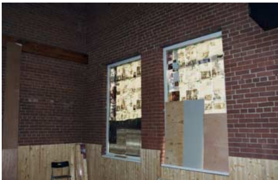
Figure 4 Interior face of South Facade
