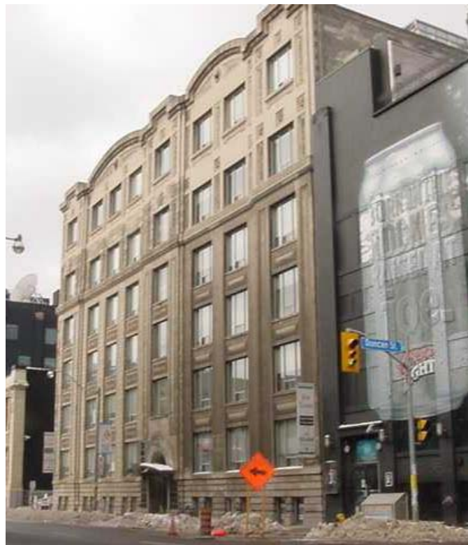
View to west, showing the principal (south) façade; the east wall (right) abuts the neighbouring building
