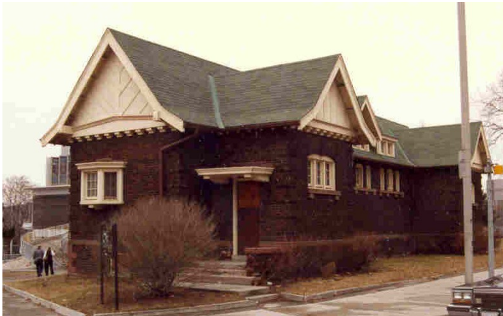
East elevation (left) and principal (north) façade (right) of Prince Edward Viaduct Public Lavatory.
