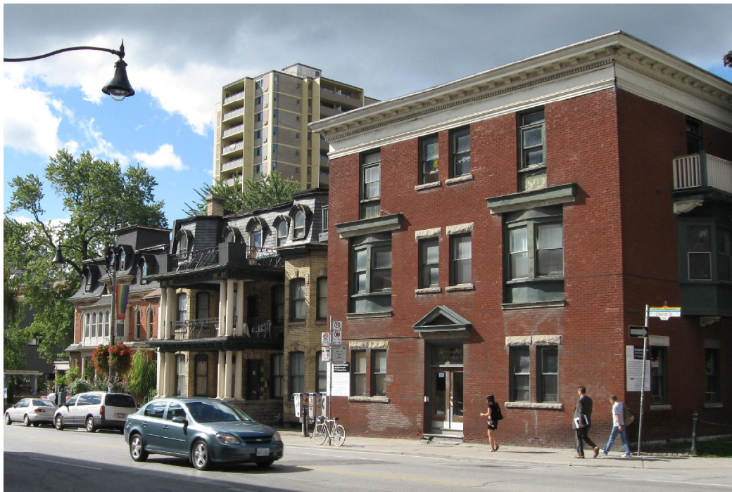
13. Contextual photograph , showing the west side of Church Street and looking south toward Dundonald Street from Gloucester Street where the Wallace Millichamp Houses (1873) stand mid-block
