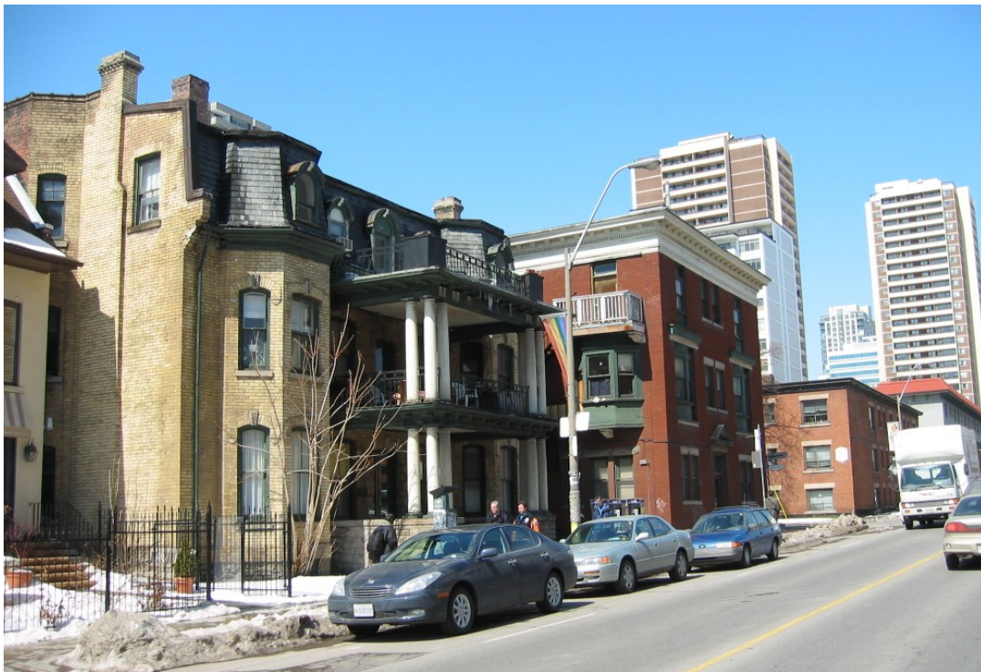
10. & 11. Photographs , showing the principal (east) façade (above) and the south elevation (below) of the Wallace Millichamps Houses (1873)
