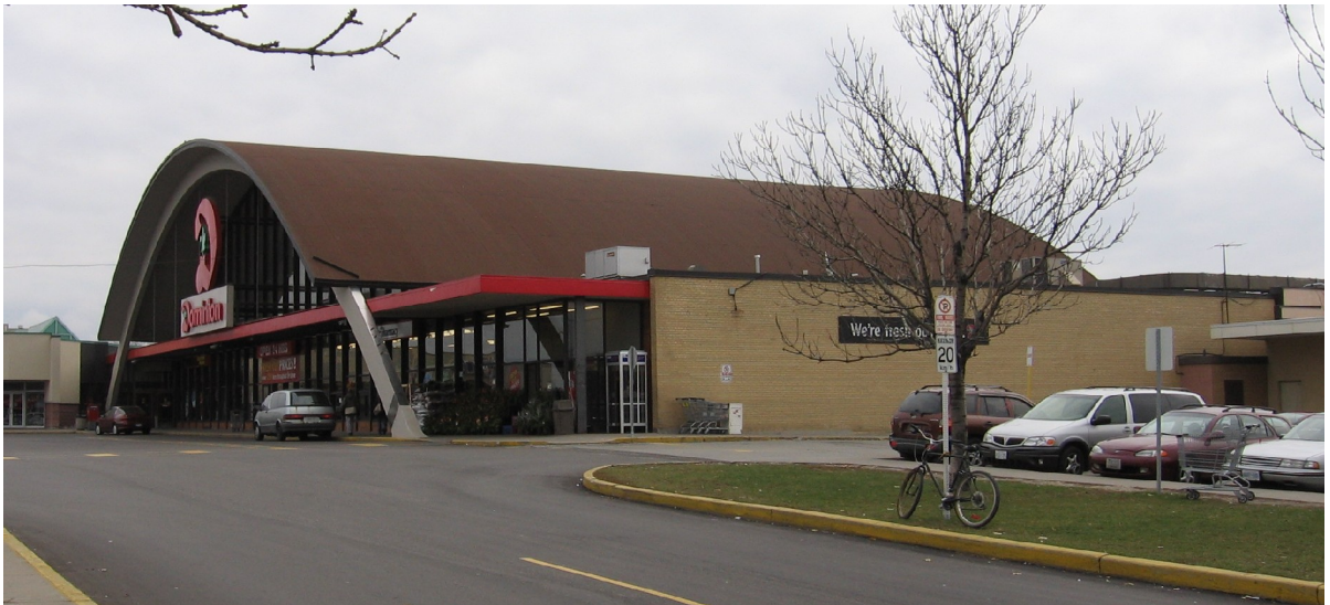
13. Photograph, Parkway Plaza, 2007 : showing the north and west elevations of the grocery store, looking east from the Victoria Park Avenue entrance to the shopping mall (Heritage Preservation Services)
