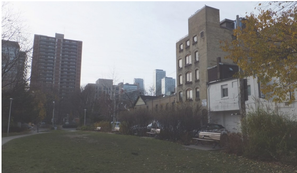
9. Current Photograph, 18 Gloucester Lane : showing the north elevation from Isabella Street with Norman Jewison Parkette on the left (Heritage Preservation Services, 2012)
