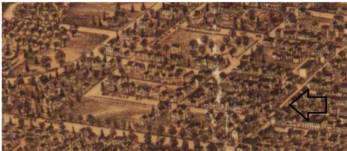
5. Gross's Bird's Eye View of Toronto, 1876 : showing the location of the subject property on the west side of Yonge Street, north of Grenville Street at the time it was occupied by the Blue Posts Hotel (the clock tower of the Yonge Street Fire Hall is depicted north, or right of the subject building)
