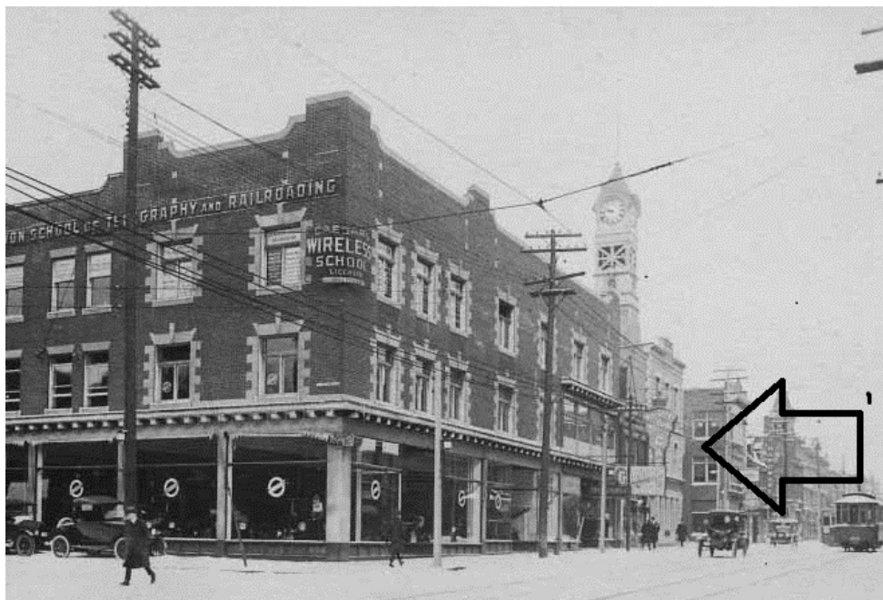
11. Archival Photograph, Yonge and Grenville Streets, 1916-19 : showing the building at present-day 480 Yonge following the addition of the third storey with the classical detailing that includes an extended pediment above the roofline (City of Toronto Archives, Fonds 1244, Item 1562)
