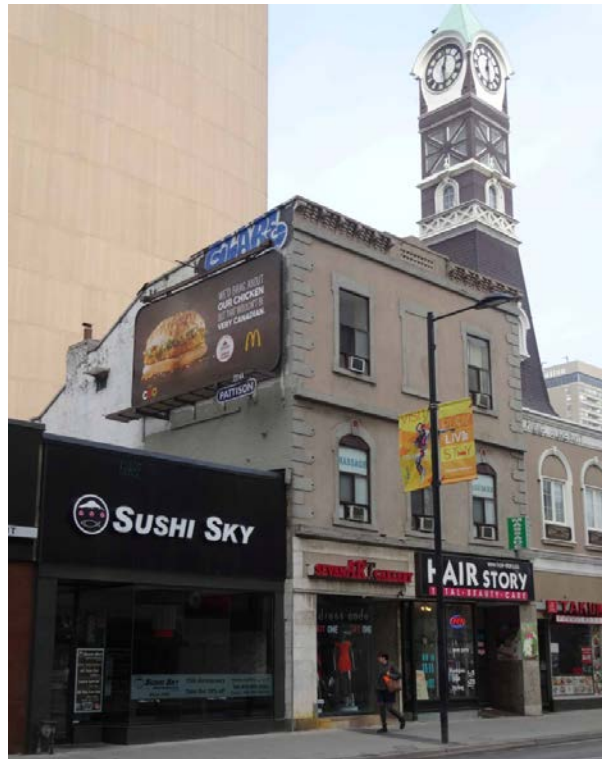
cover: east elevation; above: south (left) and east (right) elevations (Heritage Preservation Services, 2015)
