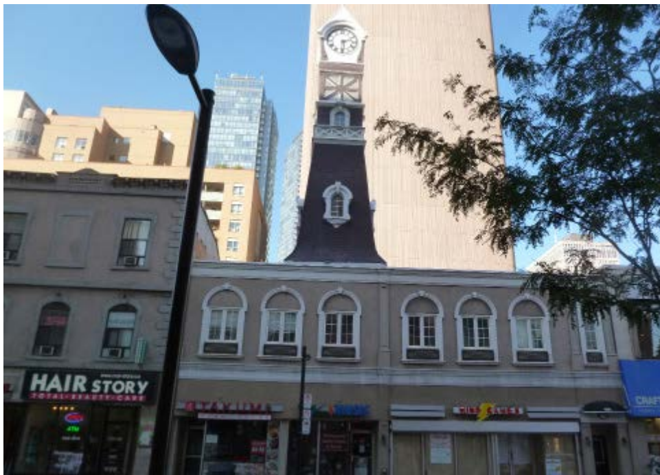
484 Yonge Street - Fire Hall Clock Tower Alterations, and HEA - 480 - 484 Yonge Street
