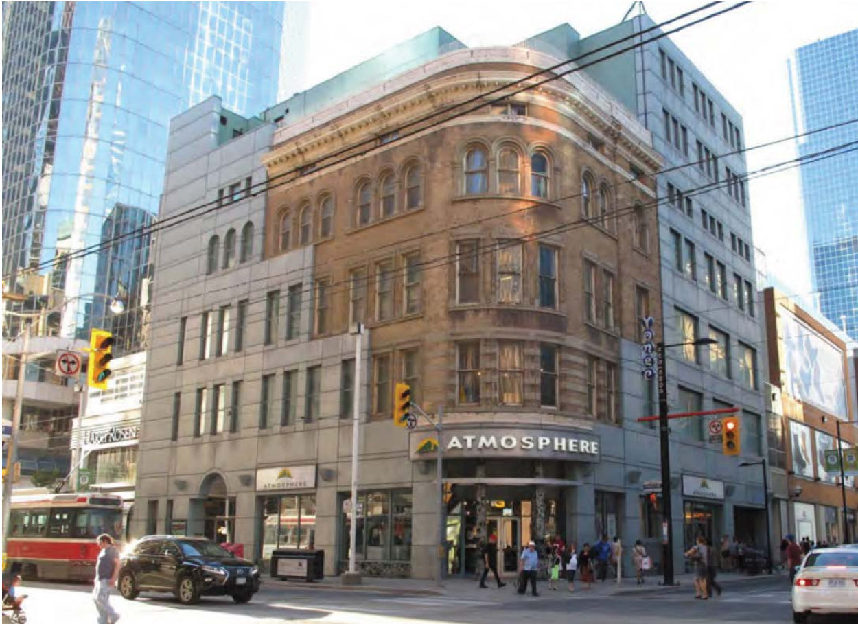
Existing Southwest Corner - 2 Queen Street West
